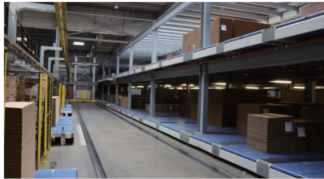
Several levels WIP
